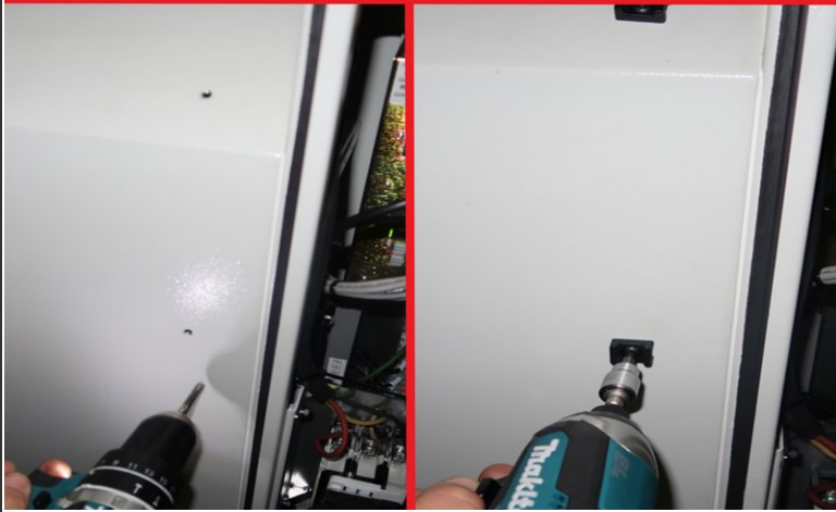
Drill, Tap, and Install Cable Tie Mounts
